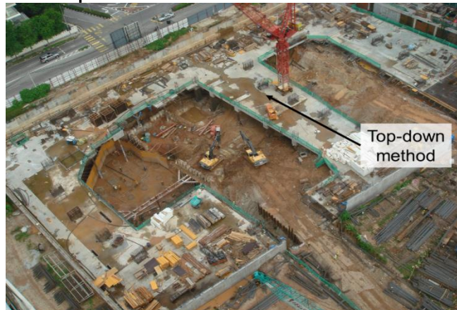
Top-down and bottom-up methods for basement construction
