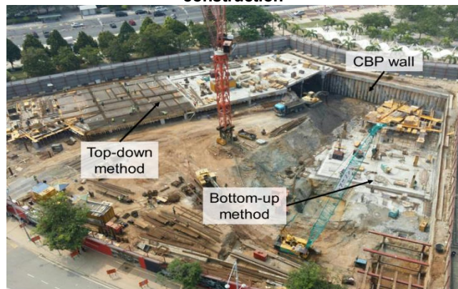
Top-down and bottom-up methods for basement construction
