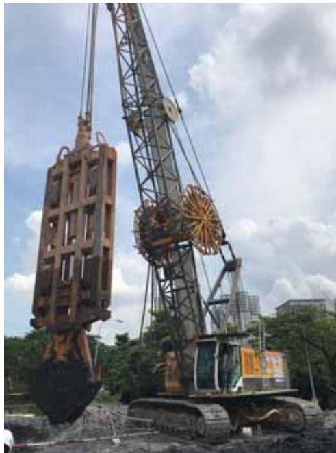
Diaphragm wall grab used for diaphragm wall construction
